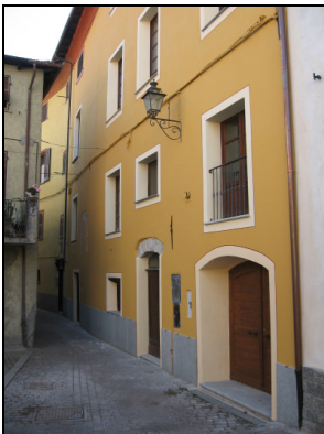
◦ Cantalupo Ligure: "Casa Spinola".
